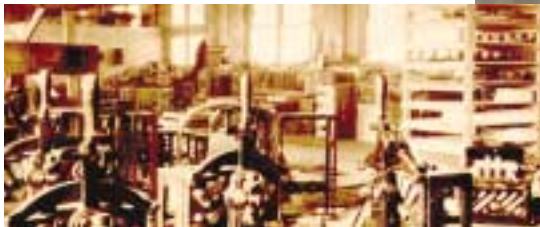
Second Floor Manufacturing
